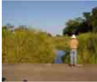
Proserpine River at Spruces Crossing (narrow culvert)
