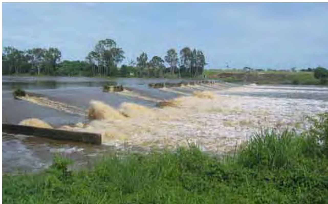
Ben Anderson Barrage overflowing in February 2008 (Photo: Tim Riseley)
