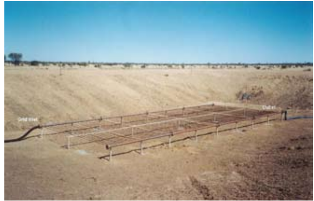
Image 1: A cooling dam prior to being filled with water
