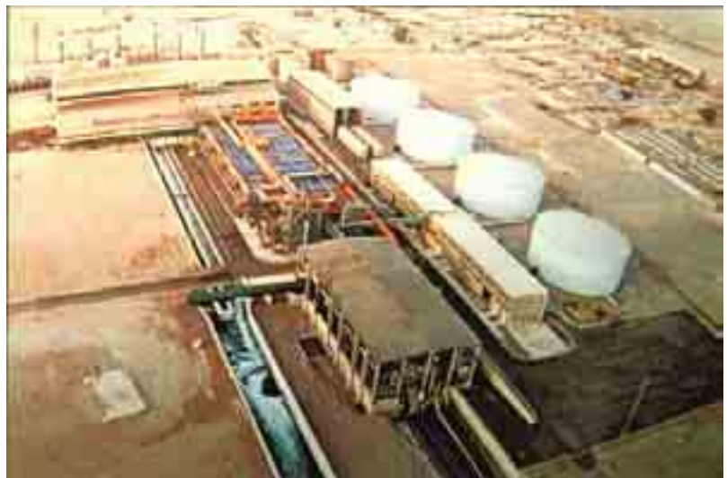
Figure B-2: Aerial view of a large MSF Distillation Plant
