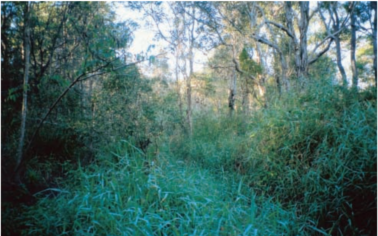
• Creek bed overgrown with vegetation: McCoy's Creek (#287)
