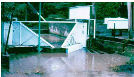
Figure 1 Flume for runoff measurement in the brigalow scrub catchment
